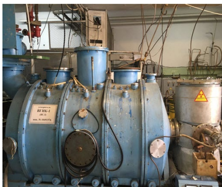
Fig. 1. Small-size accelerator VGIK-1. General view
