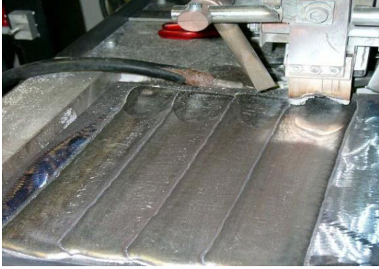
Fig. 1. Submerged arc welding using a strip electrode
