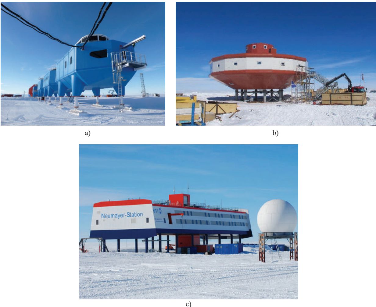
Fig. 2. Stations on high steel piles: a) Halley VI; b) Taishan; c) Neumayer.
