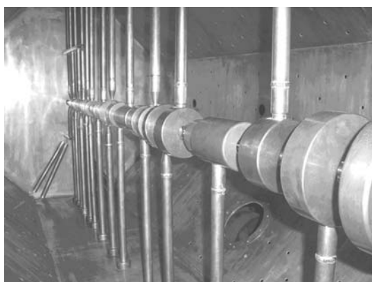
Fig.3. Accelerating structure after initial assembly
